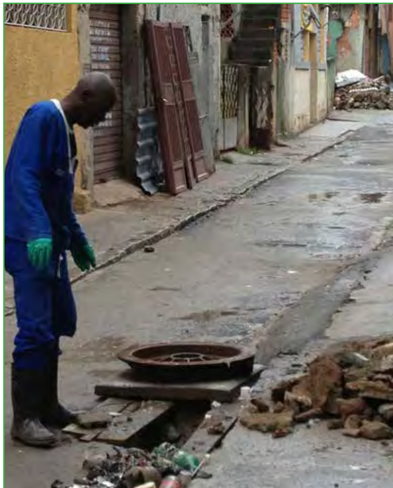
A man removes trash from a clogged sewer system.
